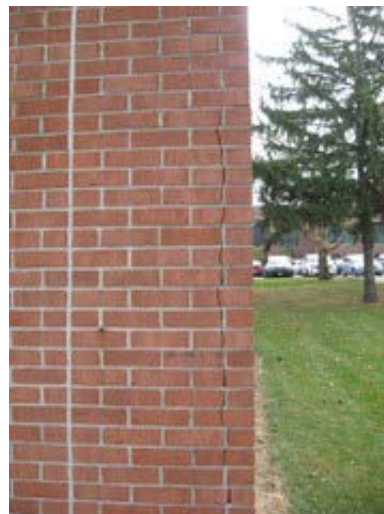
Veneer Cracks / Foundation Settlement
