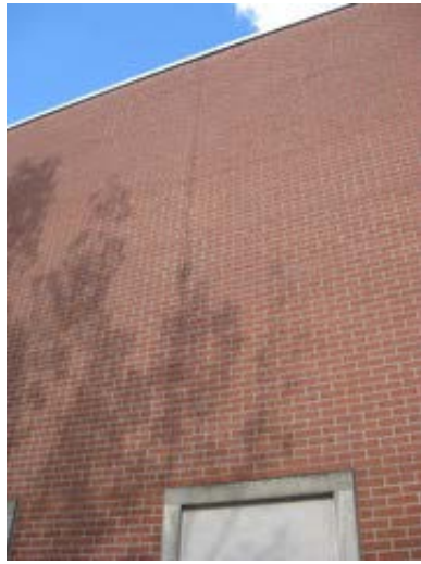
Brick Veneer and Control Joint
