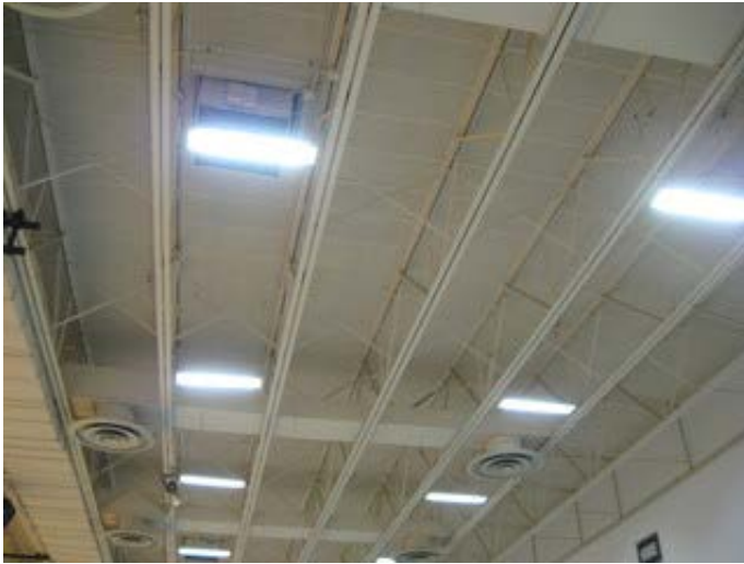
Steel Joists and Tectum Deck
