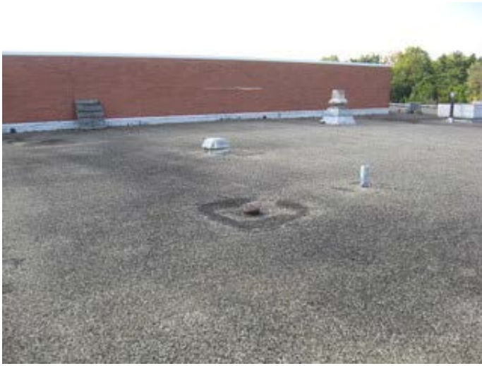
Ballasted Roof
