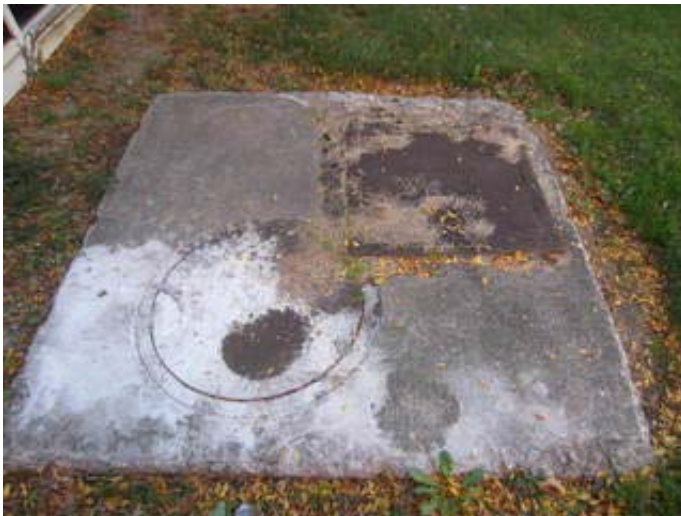
Incoming Domestic Water Service Meter Pit
