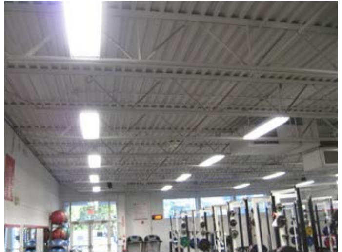
Steel Joists and Metal Deck
