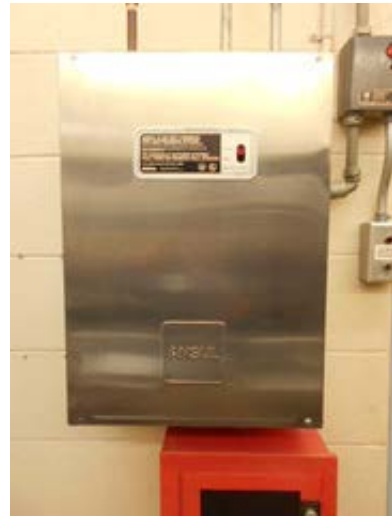
Compliant Wet Chemical Suppression System-Kitchen
