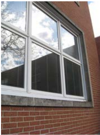
Aluminum Clad Wood Windows
