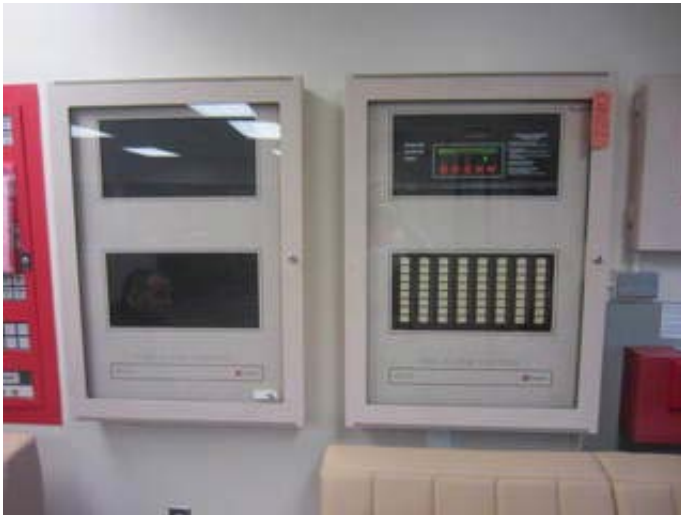
Fire Alarm System Control Panels
