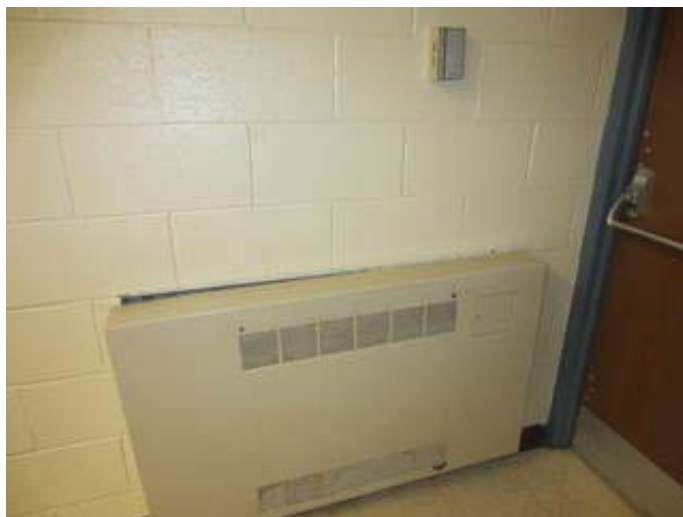
Heating Water Cabinet Heater
