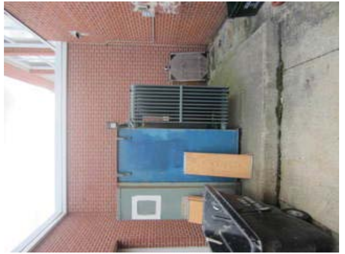
Pad Mounted Transformer
