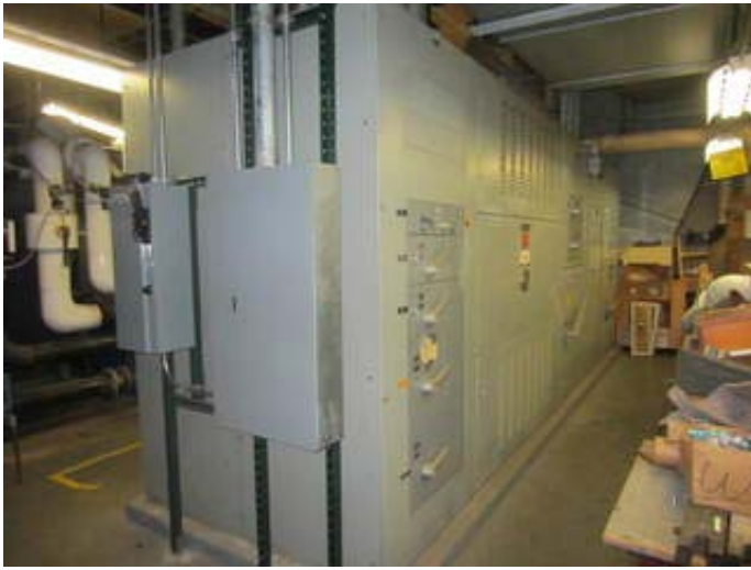
Main Electrical Distribution Panel
