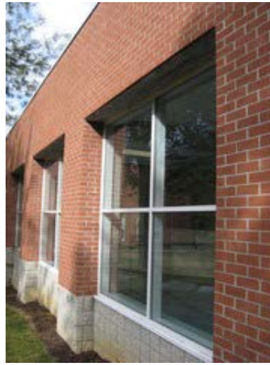
Brick Veneer and Split-Face Block
