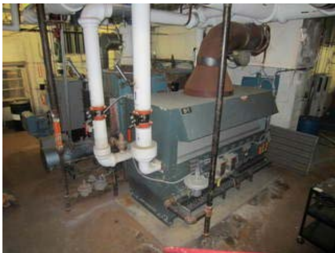
Natural Gas Fired Heated Water Boilers
