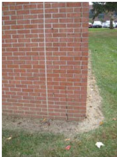
Veneer Cracks / Foundation Settlement
