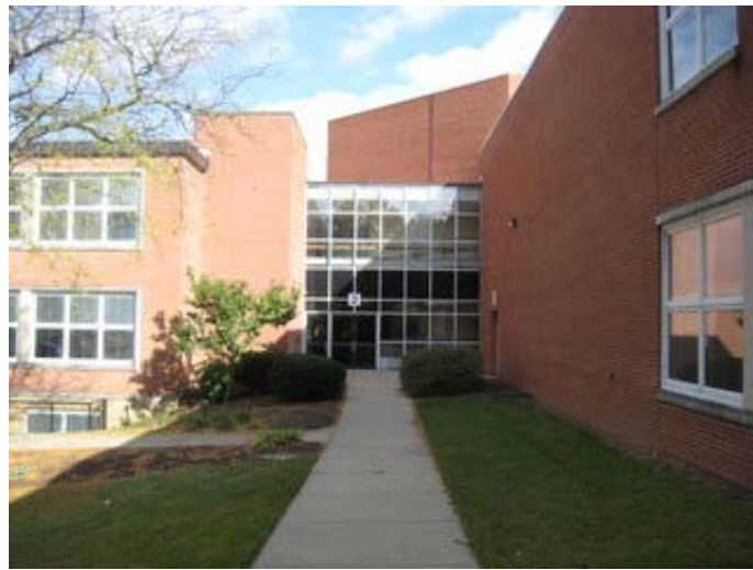
Aluminum Frame Curtain Wall
