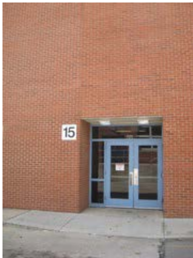
Hollow Metal Door with Transom and Sidelight
